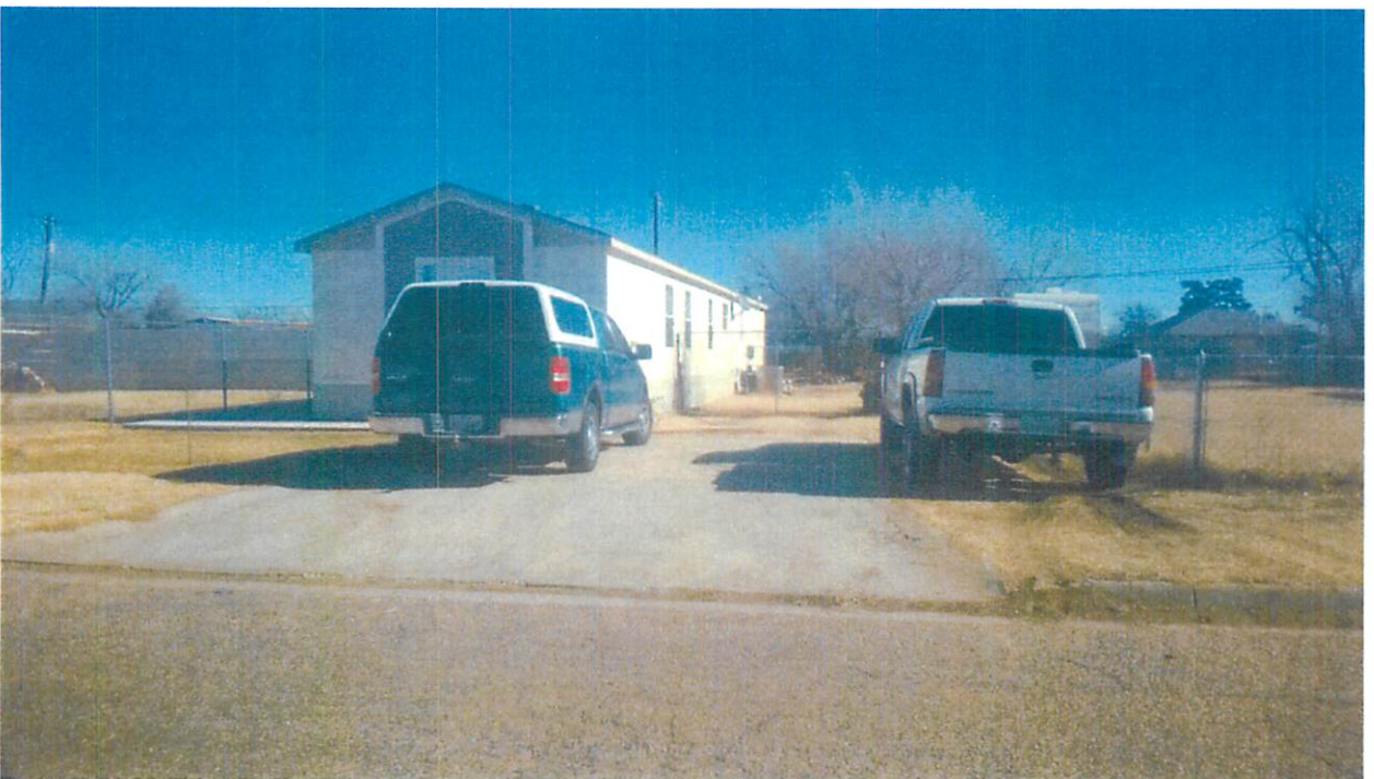
Located south of the property for consideration on South Dallas Street, SUP-171 (Approved 2013).
