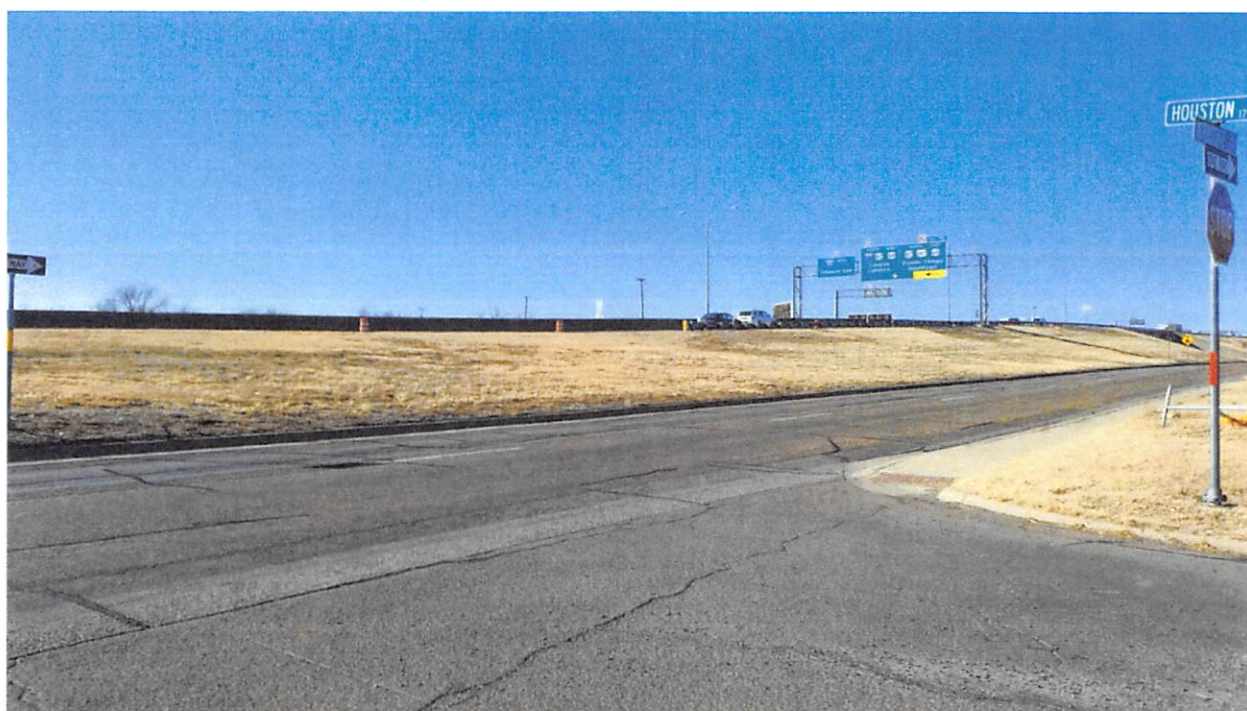
Looking Southwest from I-40 & Houston St. at adjacent Interstate 40 and access road.
