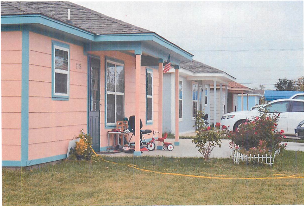
Glenwood Addition After
