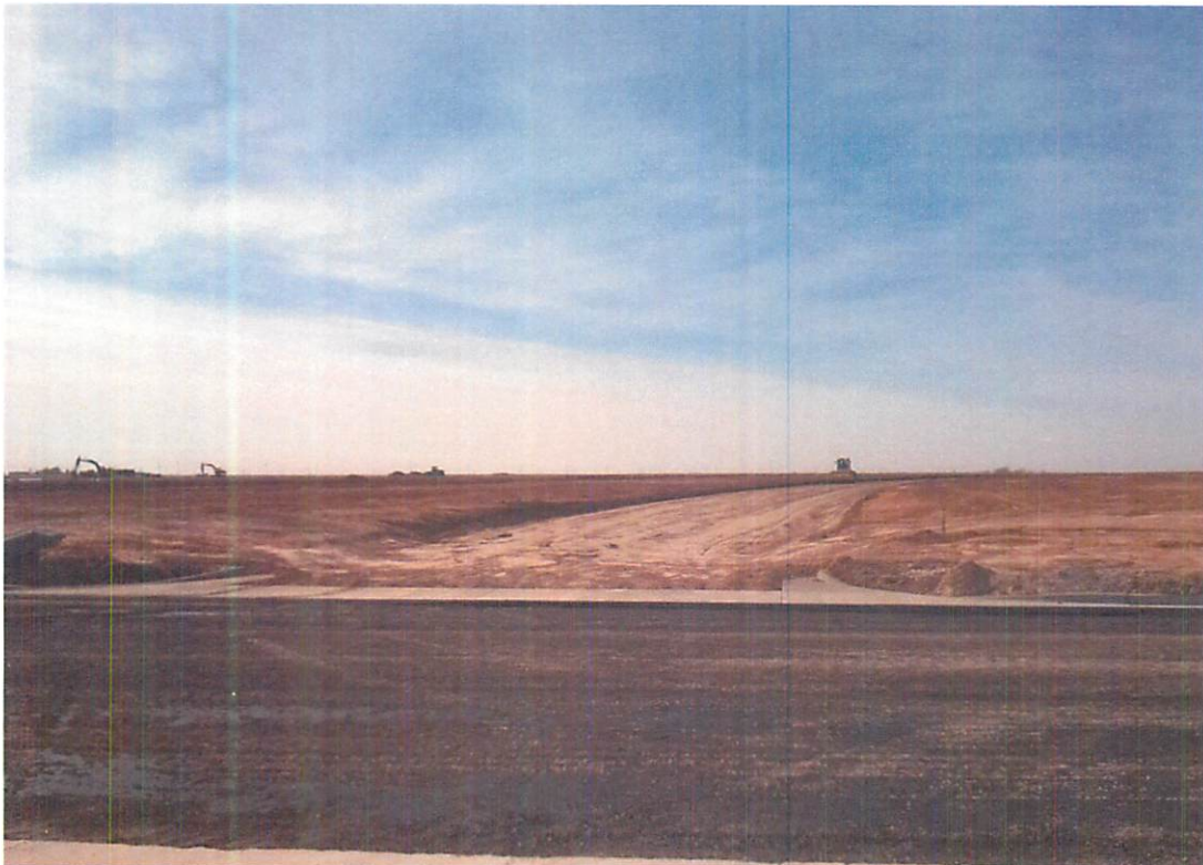
Looking west down Future Rockwood Drive from John Thomas Street
