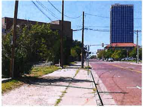
Lacking Substantial Walkway Improvements
