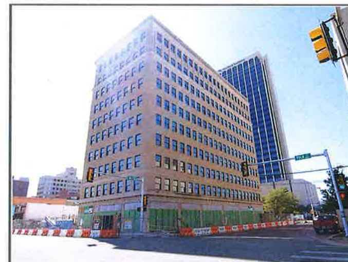
Barfield Building (During Renovation)
