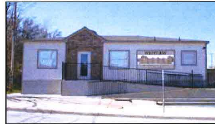
Temporary construction trailer
