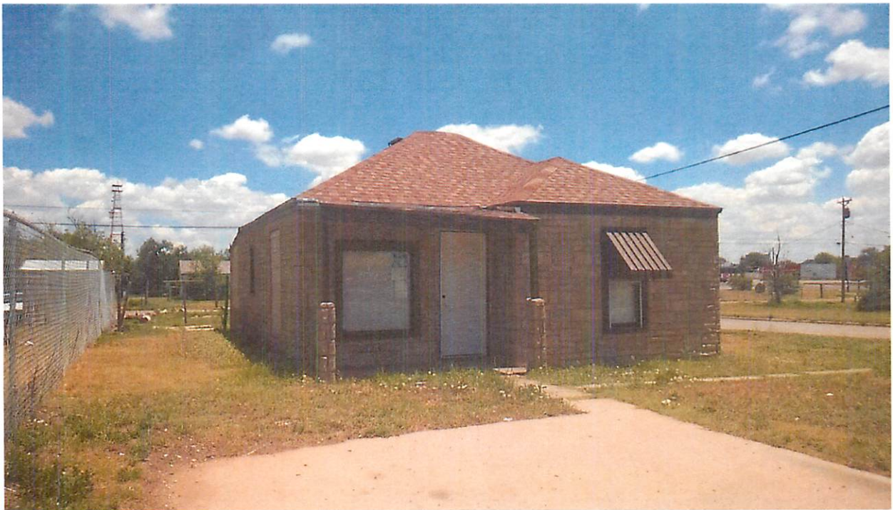
Looking southeast at the property for consideration
